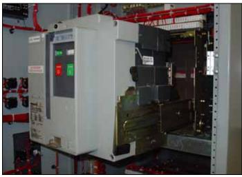
Figure 26. Switching Device Drawn Out from the Transfer Switch.
